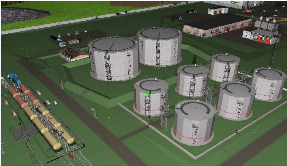
Fig.2. Discharge jetty with a park of oil-products storage
